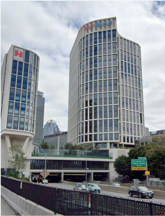
Figure 3 - The Parcel12/Lyric project with the green plaza over the Massachusetts Turnpike - © Google Maps content - Google
