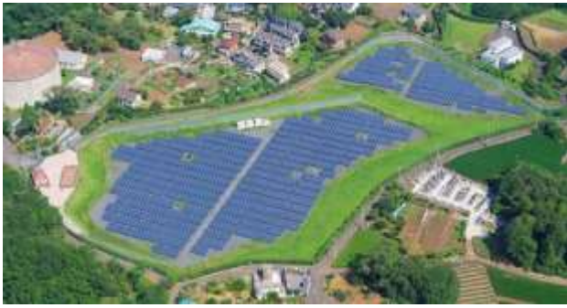
Figure 2: Mega Solar Tokorozawa
